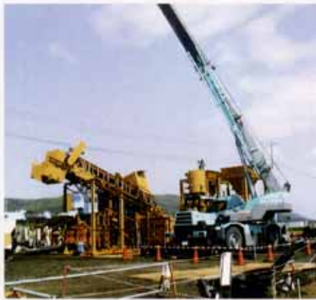
Work in progress (Solidifier Plant and Conveyance System)
